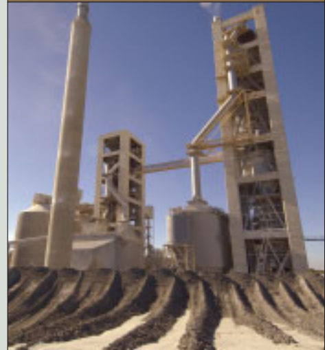
Munster cement and lime plant
