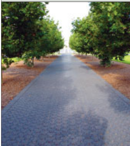
One of the many commercial paving projects supplied by C&M
