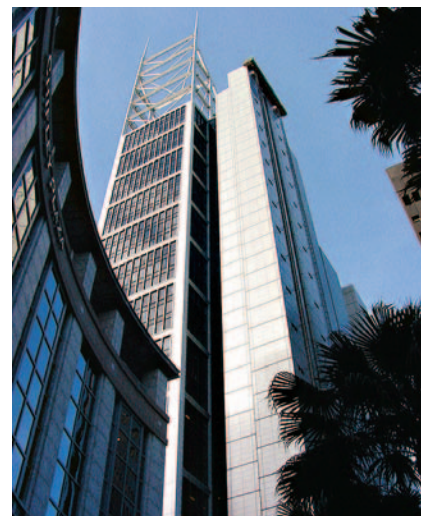
Hy-Tec's Mascot plant supplied 38000m 3 of 100Mpa high strength concrete for the 40-storey office tower at 126 Phillip Street, Sydney
