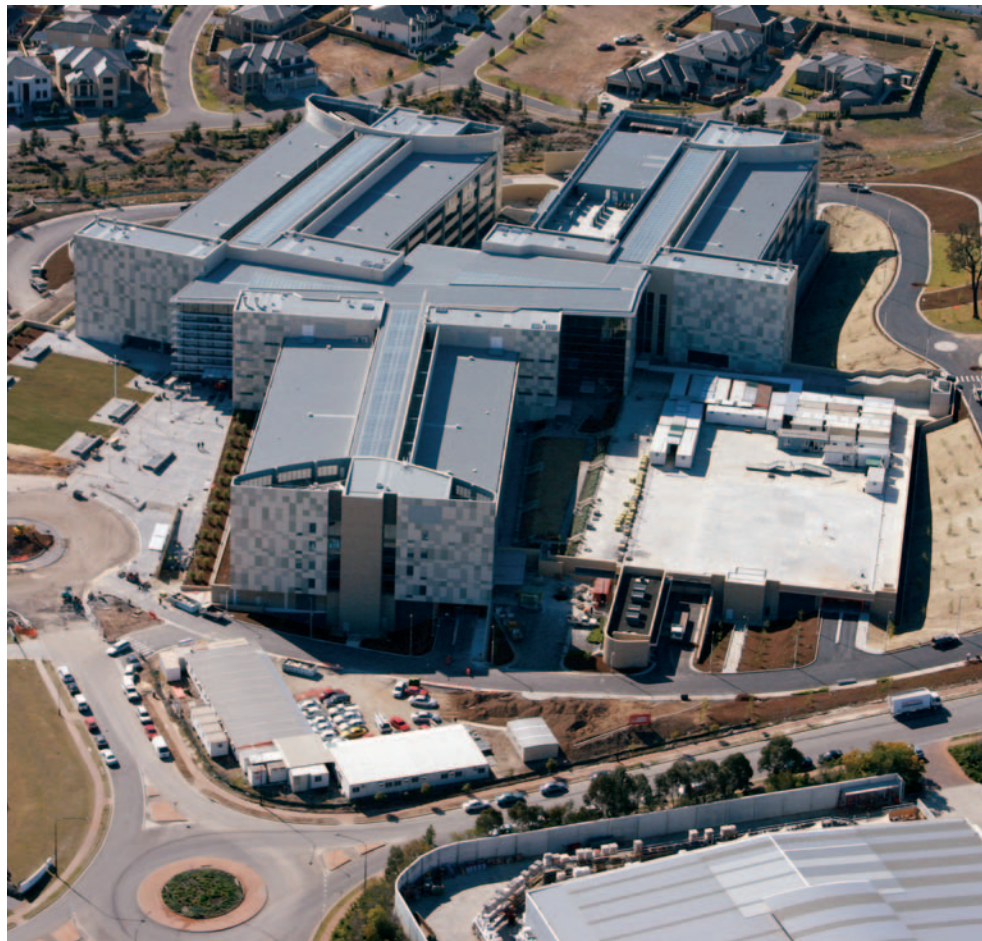
Hy-Tec supplied 40,000m 3 of varying concrete mixes over a 15 month cycle for the Woolworths Limited New South Wales corporate office
