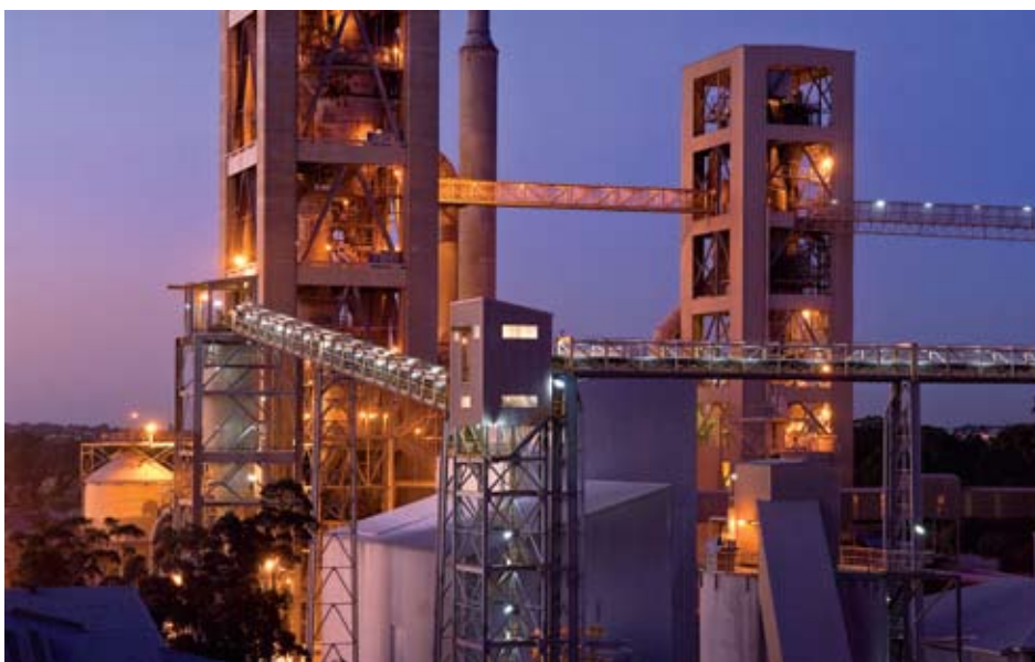
Cockburn Cement's Munster cement and lime plant
