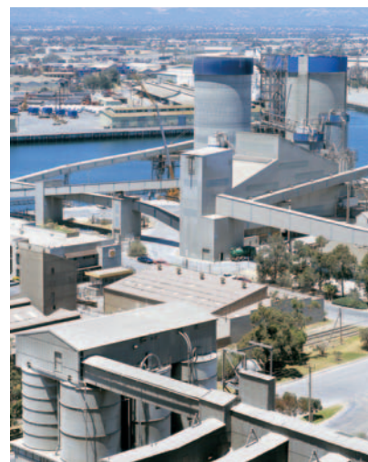
Adelaide Brighton Cement, Birkenhead plant
