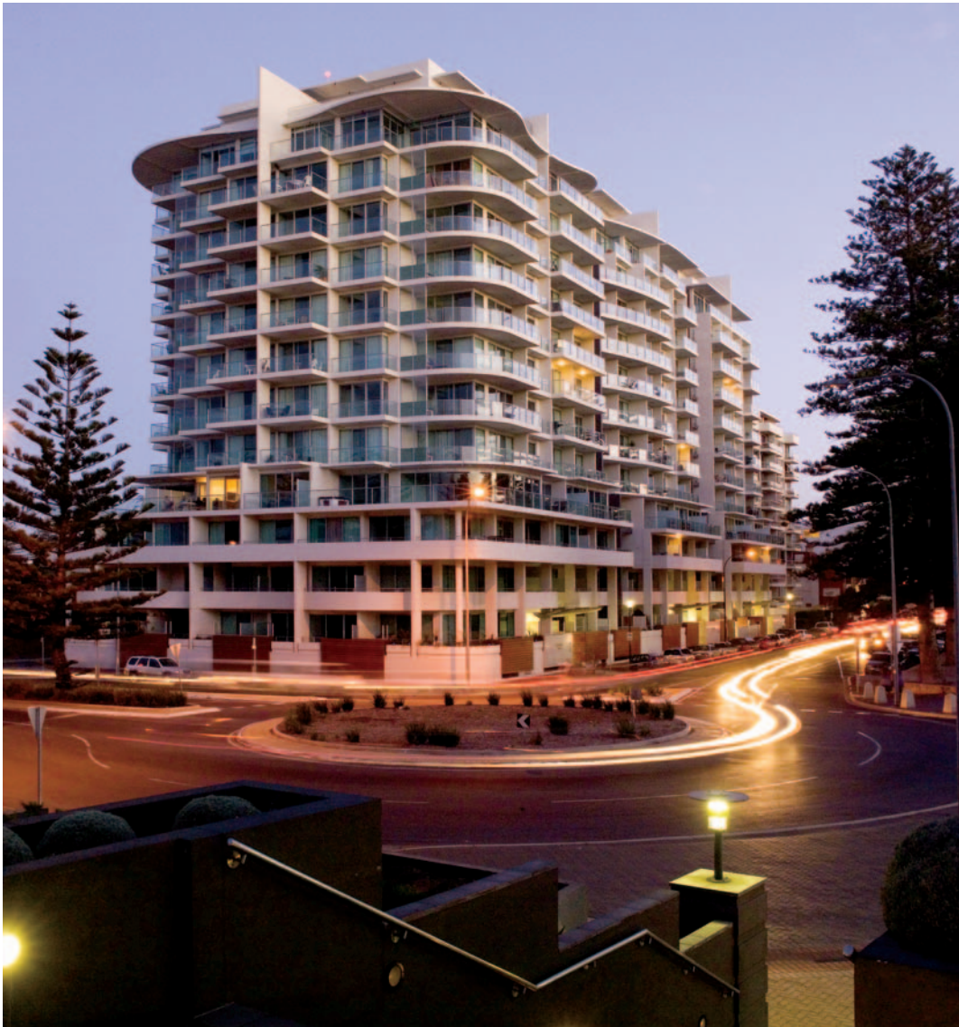
'Liberty Towers' residential complex in Adelaide constructed using precast concrete panels made from high early strength cement
