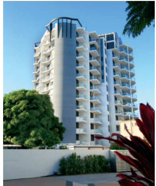
Hy-Tec's Maroochydore plant provided 32 and 40 mpa concrete and special panel mixes for the construction of the "Platinum" residential complex on the Sunshine Coast in Queensland.
