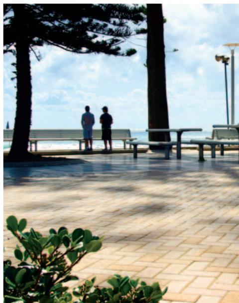
Heavy duty 'Hollandstone' pavers, custom coloured to specification and surface finished to comply with the Australian standard for slip resistance.
