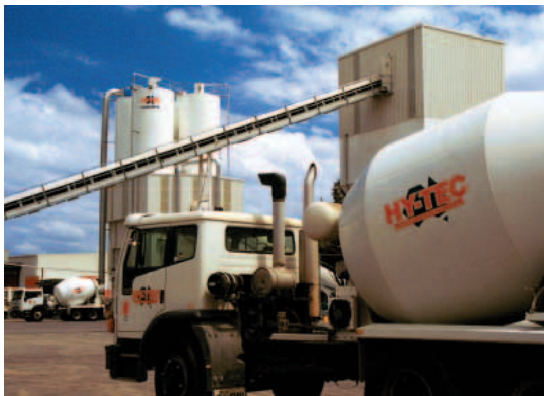
Leading edge technology has been incorporated into the recently commissioned Hy-Tec concrete plant at Mascot in Sydney
