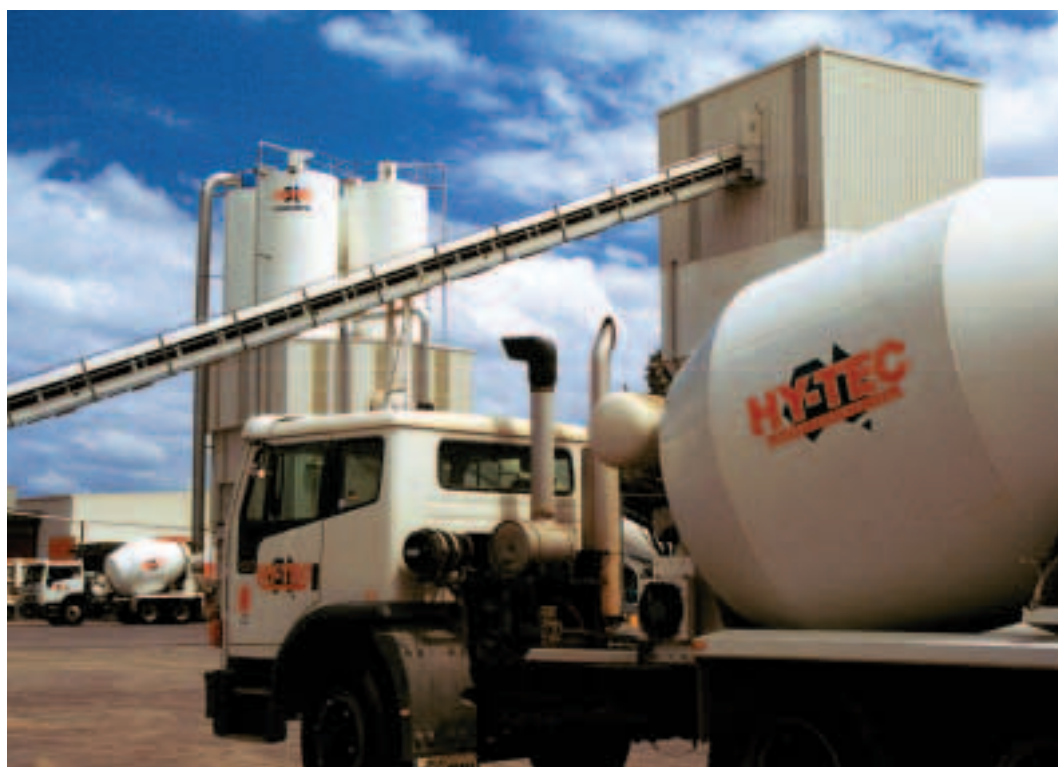
Leading edge technology has been incorporated into the recently commissioned Hy-Tec concrete plant at Mascot in Sydney
